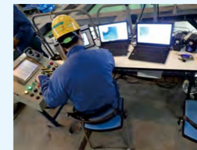
Fig.2: Remote operation for extension pipe-welding device for S/C joints
